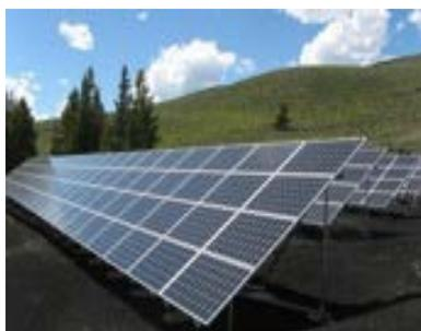
Solar panels absorb energy directly from the sun. Light from the sun hits photovoltaic or PV cells in the solar panel which convert the sun's energy into electricity.
